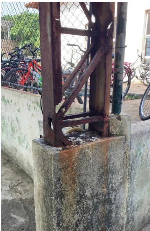
Base com concreto
