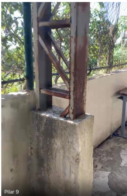
Base com concreto
