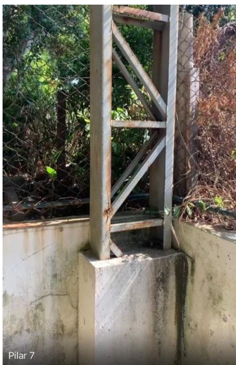
Base com concreto
